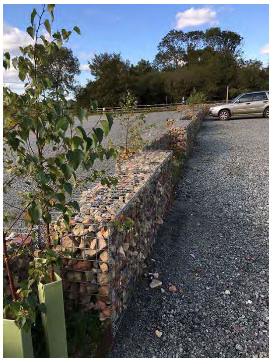
Central gabion - silver birch with biodegradable tree guard planted in 150mm deep crushed ceramics on car park base
